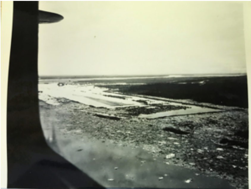
Example ice jam flood in Galena during the Spring of 1945. This runway is now protected by an earthen levee.
